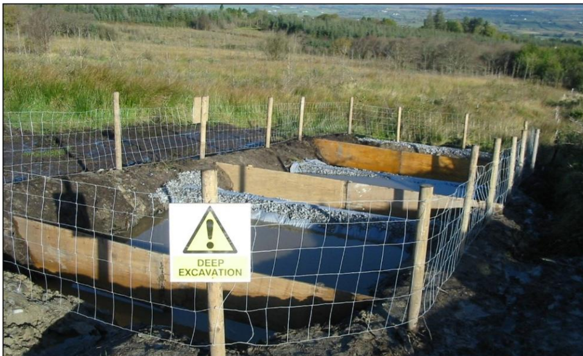
Figure 4-3: Typical Three-tiered Settlement Pond with Stone Filter
